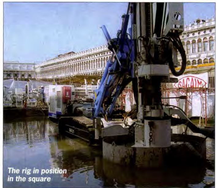
A special platform was used to distribute the nearly 22t of weight efficiently
