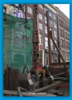
The **Grab Rotator**, a more recent development, has allowed accurate wall excavation by grab to 60 m - 80 m. In finer soils - where excavation by grab has significant advantage to the mill - **using a grab brings very substantial cost savings.**
