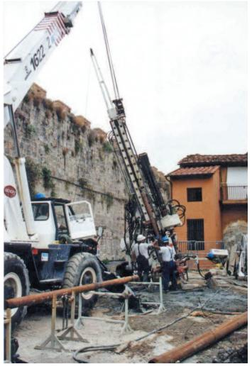
Temporary rigging trestle used to attach a backstay to the Tower, to prevent potential movement of the Tower during restoration operations.
