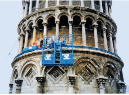
Steel cables sheathed in Teflon being positioned and tensioned around the first story cornice with a specially-designed device.
