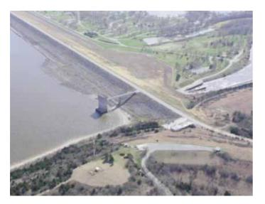
From the outcome of this field test and the preconstruction services provided by Treviicos South, the USACE completely re-designed the downstream stabilization selecting the use of the slurry wall technology to build some 350 self hardening cement bentonite walls, 45 ft long, 4 ft wide and 70 ft deep, that were installed perpendicular to the axis of the dam.
