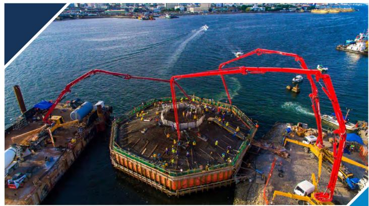
In order to shorten the time and increase the accuracy when installing the steel cages, special tools and equipment were studied and developed by Trevi's technical team in Italy and in the Philippines. The H.C.T.S. (Hydraulic Catapult Trevi System) was developed and is being implemented in the project.
