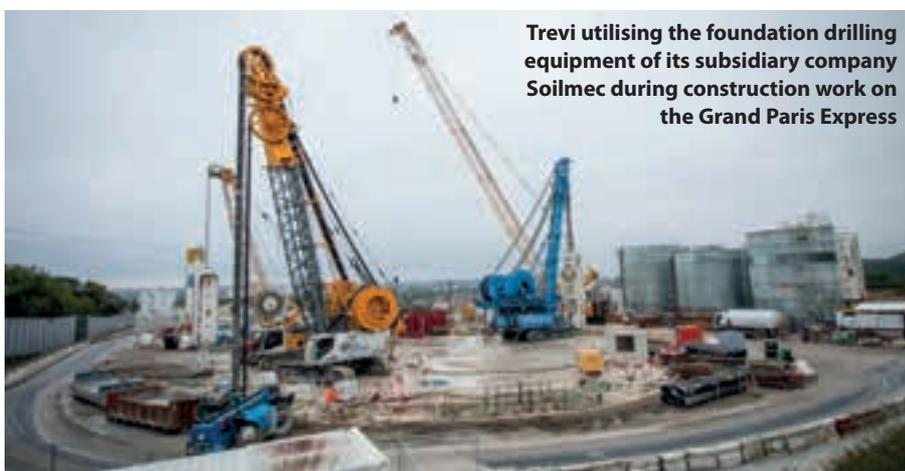
Trevi utilising the foundation drilling equipment of its subsidiary company Soilmec during construction work on the Grand Paris Express
