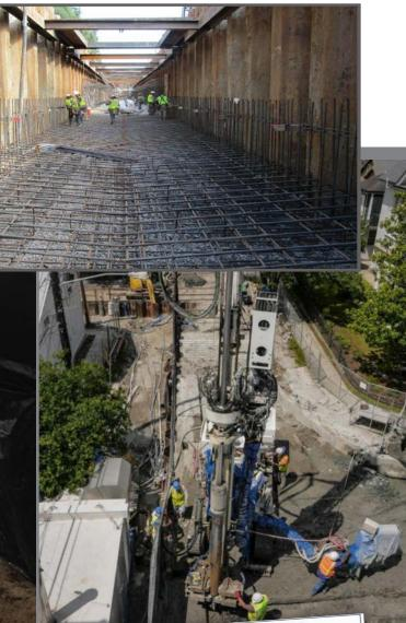
coring to be executed on 5% of the installed columns. At intervals of 3.0 ft. of vertical treatment, soil-cement mixture was tested for unconfined compressive strength (UCS) and hydraulic conductivity (HC) and the 28-days results needed to comply with the minimum design criteria of 100 PSI and  $1x10^{-6}$  cm/s respectively.
