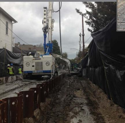
The elliptical jet grouting solution proposed for the SELA-22 in Uptown New Orleans proved to be efficient and effective in resolving the constructability and engineering challenges it had been designed for. Notwithstanding this was the first time this technology was used in the U.S., and in particular in mostly cohesive soils, it showed high reliability and outstanding quality of the final product.
